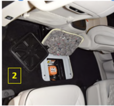
Second: Unbolt the cover panel over the Service Disconnect.
